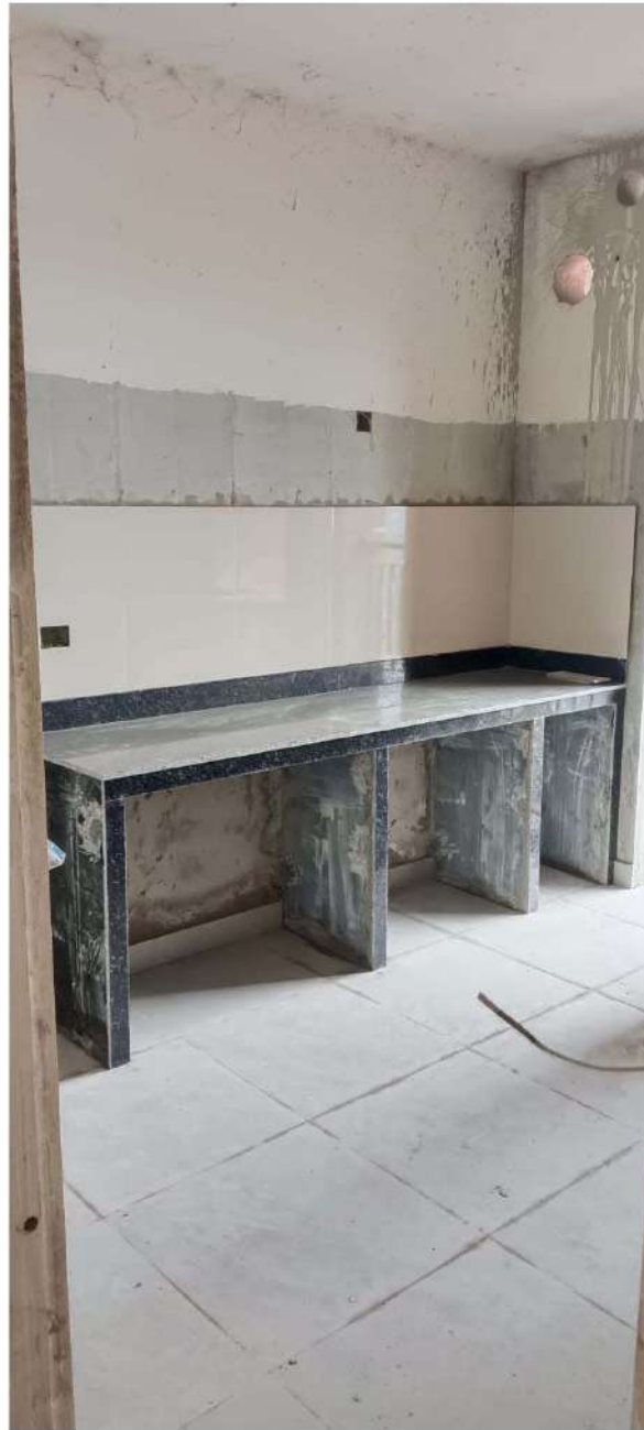
Tower 2 Kitchen Counter tiles fixing work in progress
